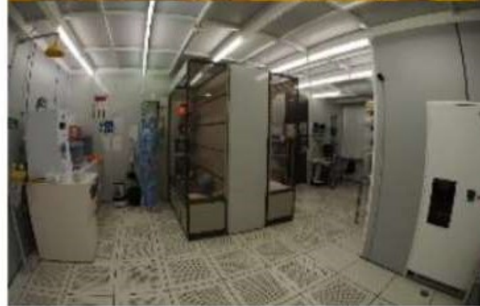
500 m 2 (250 m 2 class 100) MEMS and CMOS Clean-Room
