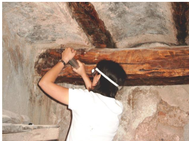
Fig. 2: On site investigation training course, (Valencia_Spain_2008);
