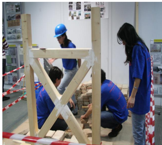
Fig. 3: Construction of a model timber house, (Reggio Calabria, Italy_2007);
