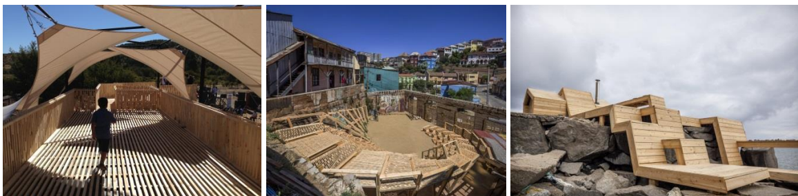
Fig. 1. Three projects by the SCS studio; Left: Community center in Pumanque, Chile, Center: “The Wave”, amphitheater in Valparaiso, Chile, Right: “The Bands”, sauna in Lofoten, Norway.
